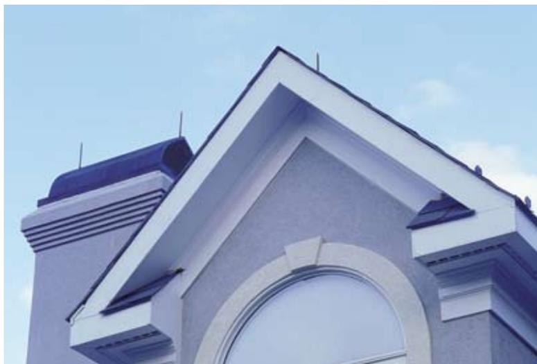
*A lightning protection system is intended to last the life of the structure it protects and typically only requires maintenance if a home is changed structurally or mechanically. Such changes might include a new roof, an addition, a new electrical service or the installation of a satellite dish.*
